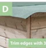
Neaten & cut excess felt
