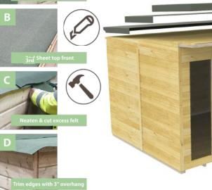
**17c.** Trim down excess felt with a stanley knife. Remember to overlay the 1st felt to avoid rain leaks.
