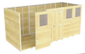
13a. Place the final front panel as shown (Below) to complete the outer framework. Then adjust and screw down the panels to the shed floor to make the build secure. This requires an extra 3x Screws.
