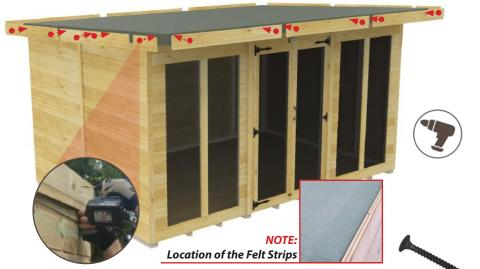
**18c.** Felt Strips must be same height as roofing felt to allow rain water to run off. See Diagram on the right.
