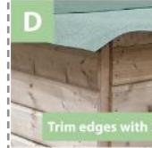
Neaten & cut excess felt
