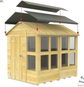
**15c.** Trim down excess felt with a stanley knife. Remember to overlay the 1st felt to avoid rain leaks.
