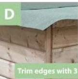
Neaten & cut excess felt
